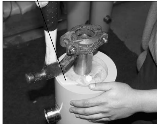
Figure 8-14 Remove Access Cover Position II
