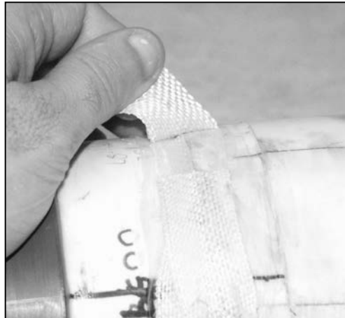
Figure 8-6 Remove Fiber Glass Tape
